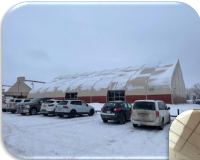
PICTURE 3 – SPRUNG STRUCTURE
