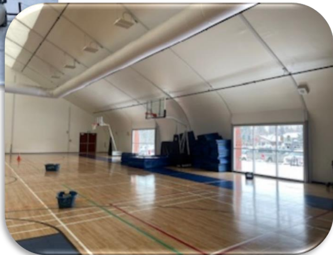
PICTURE 4 - SPRUNG STRUCTURE
